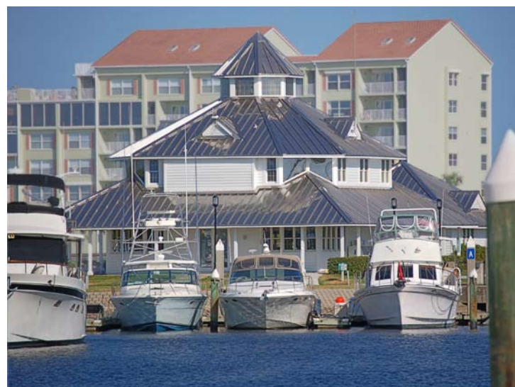
Halifax Harbor Marina in Daytona, FL • Series 300 System in Stainless Steel
