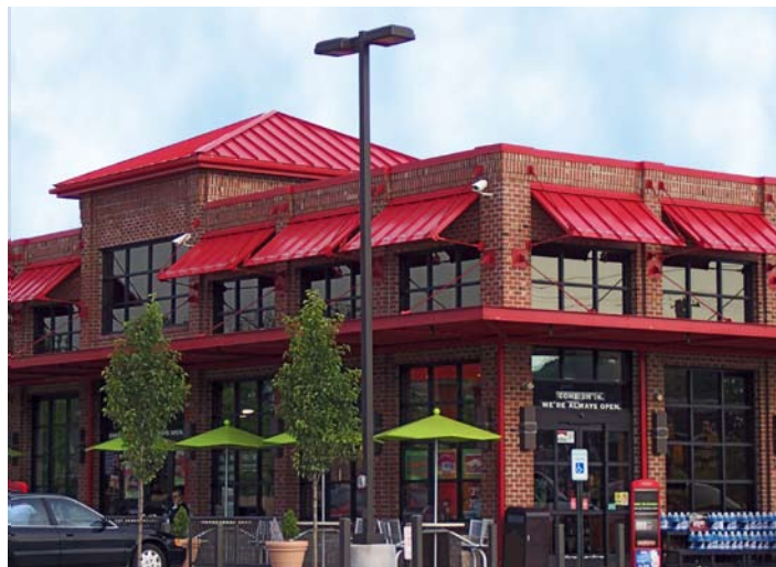
Sheetz Store in Altoona, PA • Snap-Lok System in Heritage Red
