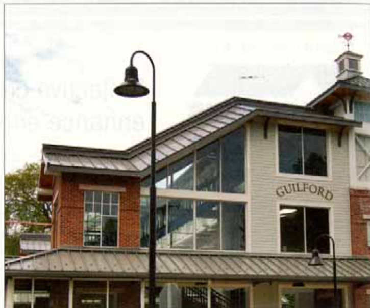
Symmetrical seam roof on Shoreline East Railroad Guilford Station shelters daily commuters in Guilford, Conn.
