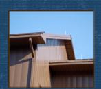
The FW Series wall and soffit system is an attractive, cost-effective flush metal panel. Its interlocking legs conceal fasteners and improve strength and flatness.
